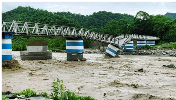
Dudhia iron bridge collapsed due to heavy rain in Darjeeling
